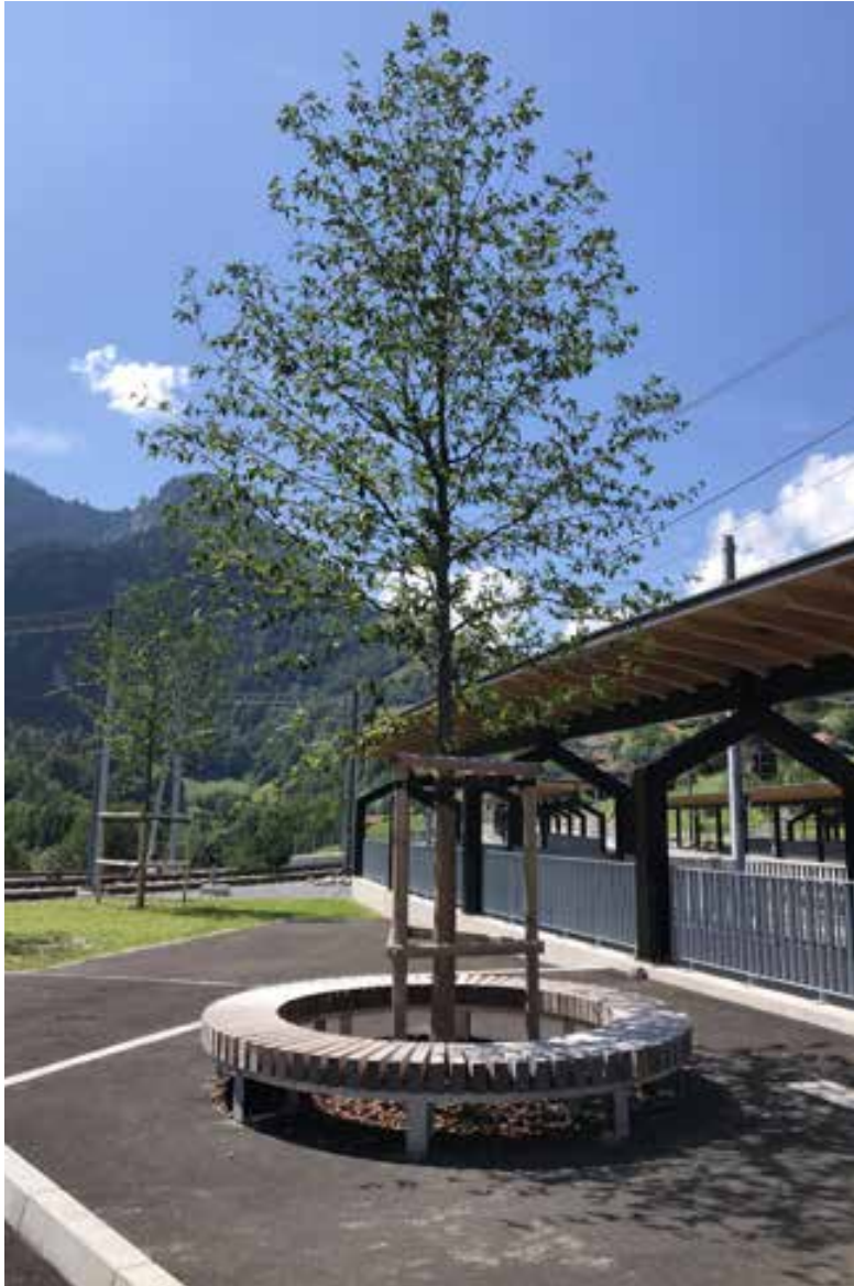
Montbovon, Switzerland 8 mm hot-dip galvanized steel structure. Seat in exotic wood moabi.
